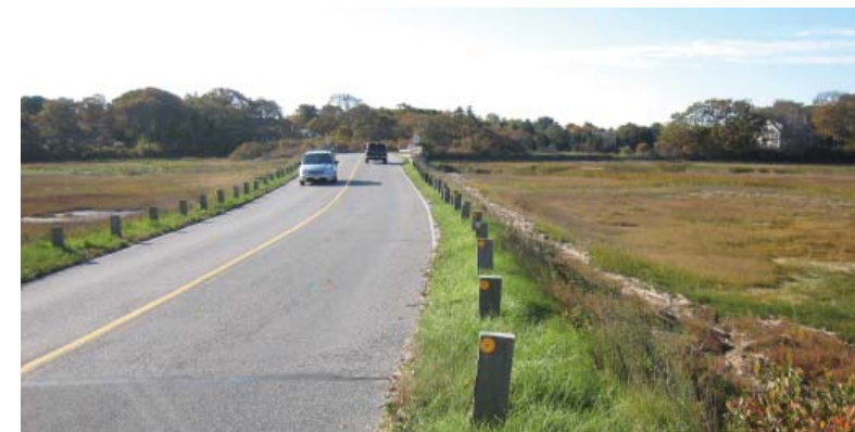
Road crossing salt marshes at Bridge Road in Eastham.
