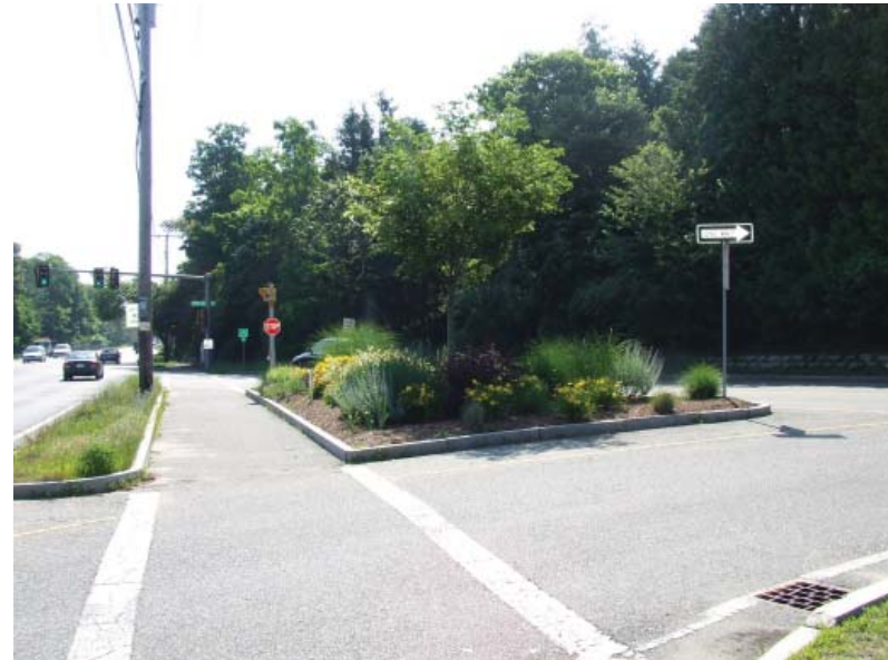
A raised median guides traffic and protects pedestrians on Phinney's Lane in Barnstable.
