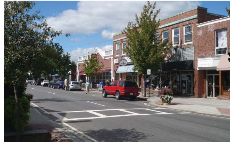
Curb extensions narrow pedestrian crossing on Main Street, Hyannis.
