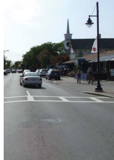
Lighting at crosswalk on Main Street in Hyannis.
