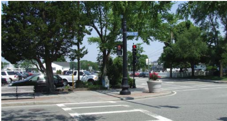
Curb extensions reduce turning speeds and protect pedestrians in Hyannis.
