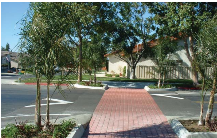
Arrows to indicate raised pedestrian crossing.
