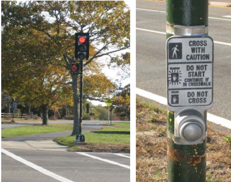
Pedestrian signal crossing and detail at Route 6 in Eastham.
