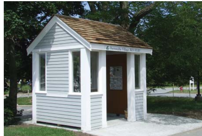
Bus shelter in Barnstable Village.
