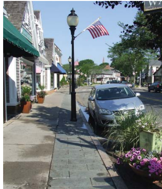
Stone and concrete sidewalk in Falmouth.
