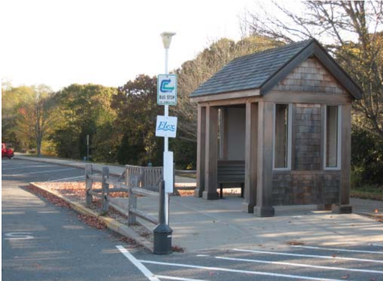
Bus pull-out and shelter at Salt Pond Visitor Center, Cape Cod National Seashore.
