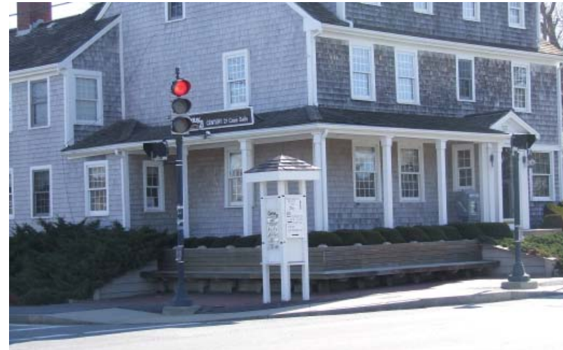
Sandwich village improvements at Route 6A and Jarves Street.
