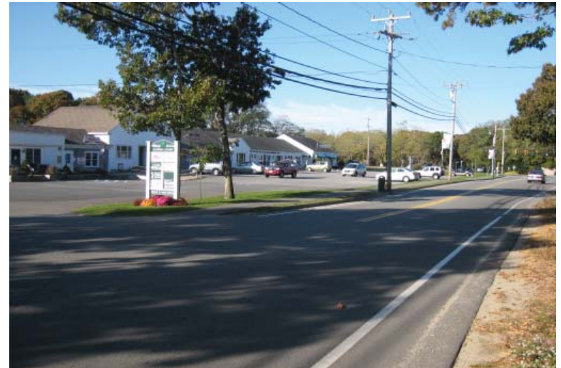
Multiple curb cuts were consolidated into one access point on Bracket Road in Eastham.
