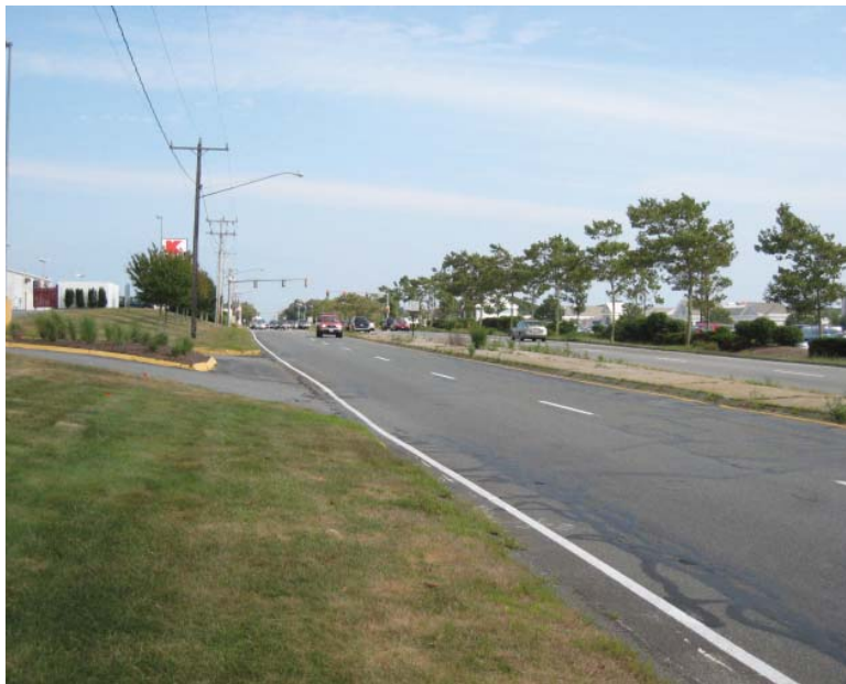
Route 132 in Hyannis - two travel lanes in each direction, divided by a raised median strip, with large scale commercial uses and deep setbacks.
