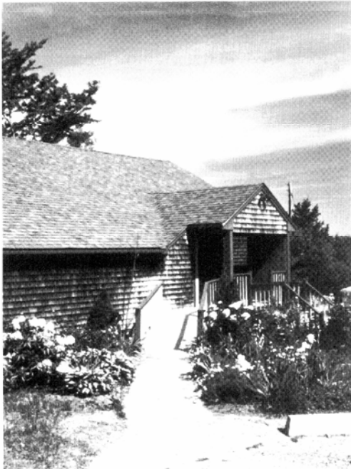
A well designed, accessible entry
