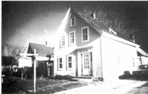
Residence converted to commercial use with an apartment above
