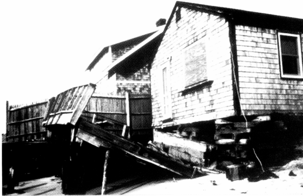
Storm damage to poorly sited home
