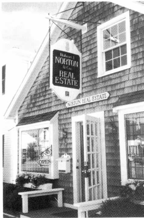
These signs are small, complement the building and are compatible with surrounding materials
