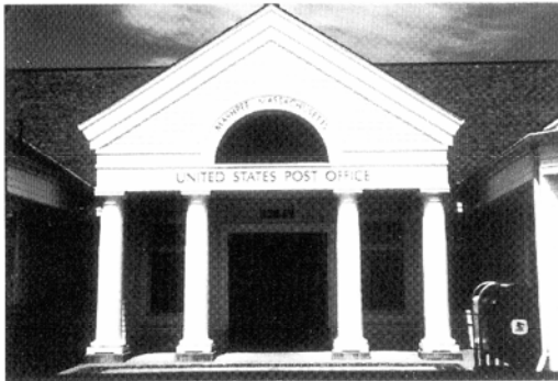
Encourage the construction of civic buildings like this one in Mashpee Commons
