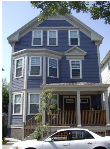
Towns over Flats
