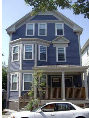
Towns over Flats
