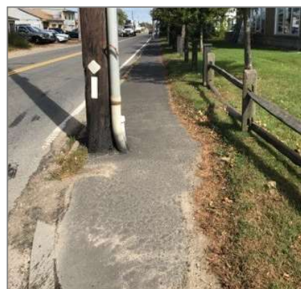
Figure 6. Existing Condition of Pedestrian Facility
