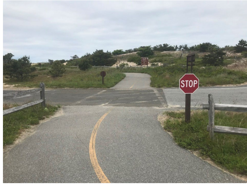
Figure 52: Path Approach to Crossing (Facing North)
