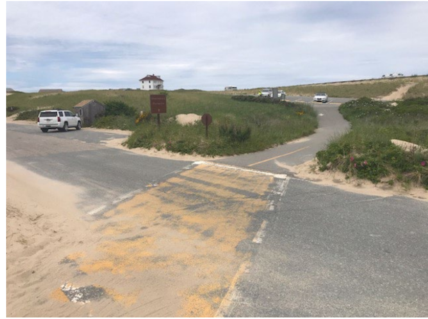
Figure 50: Path Approach to Crossing (Facing Toward Parking Lot)
